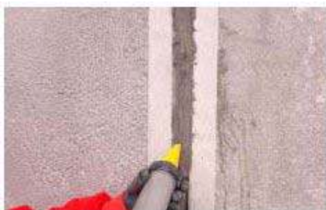
Application of MAXJOINT® ELASTIC
