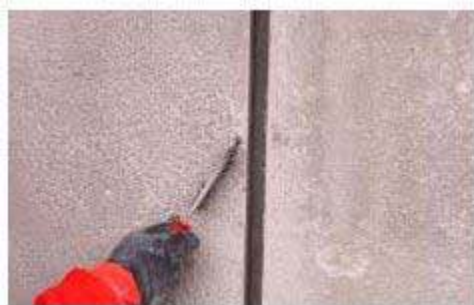
Preparation and cleaning of joint
